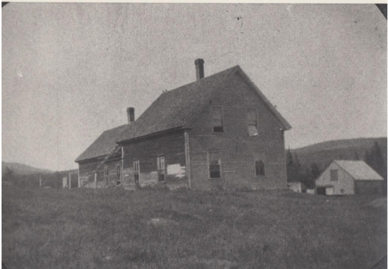
Figure 15. View north rear of Wheeler place. Note: post office, 1 st floor, right side, Wheeler barn in background.
