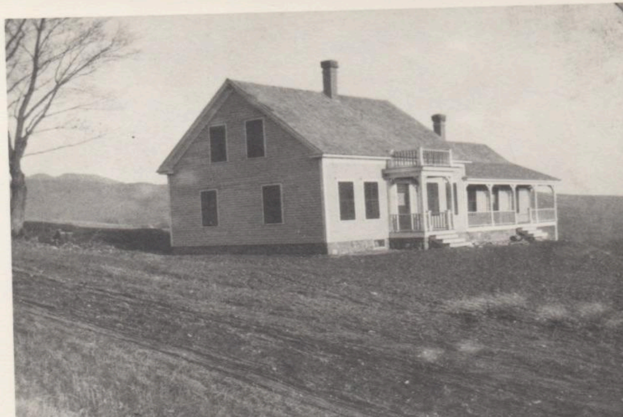
Figure 36. Historic views of the Tosier farm. Upper: Original farmhouse. Lower: Farmhouse showing early 20 th century alterations.
