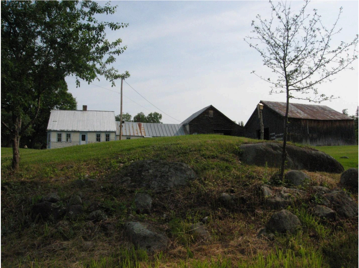
Figure 17. Northerly dam abutment of the True-Hinkley Mill.
